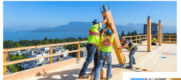
This 18-story tower, a student residence in Vancouver, was world's tallest wood building (as of 2018). Completed in <70 days using prefabricated components – four months ahead of schedule.
